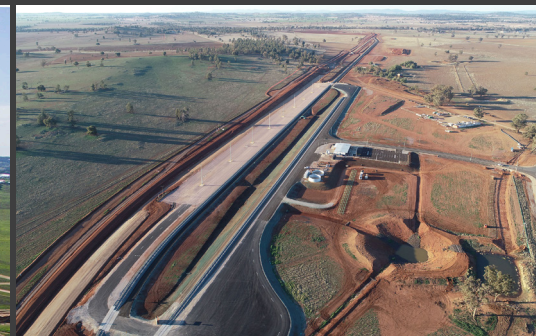
Parkes Logistic Terminal
